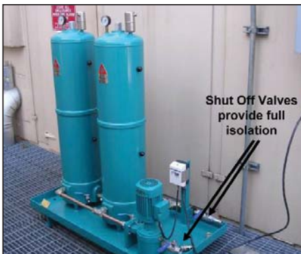
Figure 1: C.C. Jensen's varnish removal skid has four replaceable cellulose filters, each capable of removing 8 lbs of varnish
